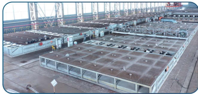
大单式环式炉 18室 Large Single-chamber Rotary Furnace, 18 Chambers
